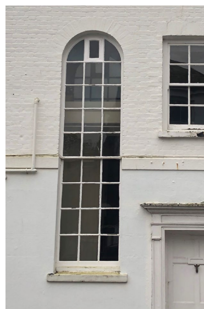
Tall arched window, Albert Quay
